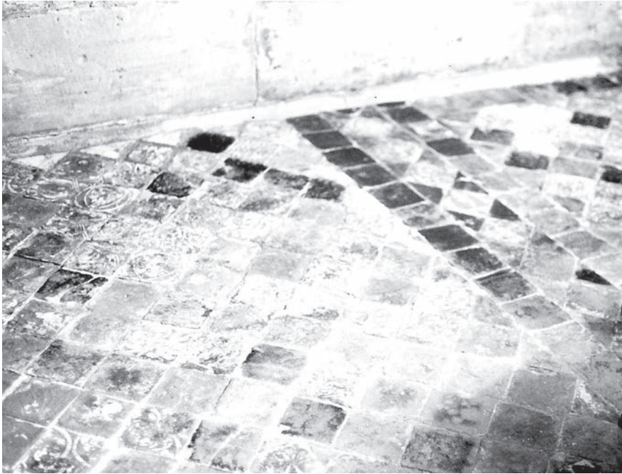
Figure 1.3 Part of the thirteenth-century floor in the suite of guest chambers in Guy's Tower, Warwick Castle, showing the diagonal format with double tramlines of inserted tiles.
